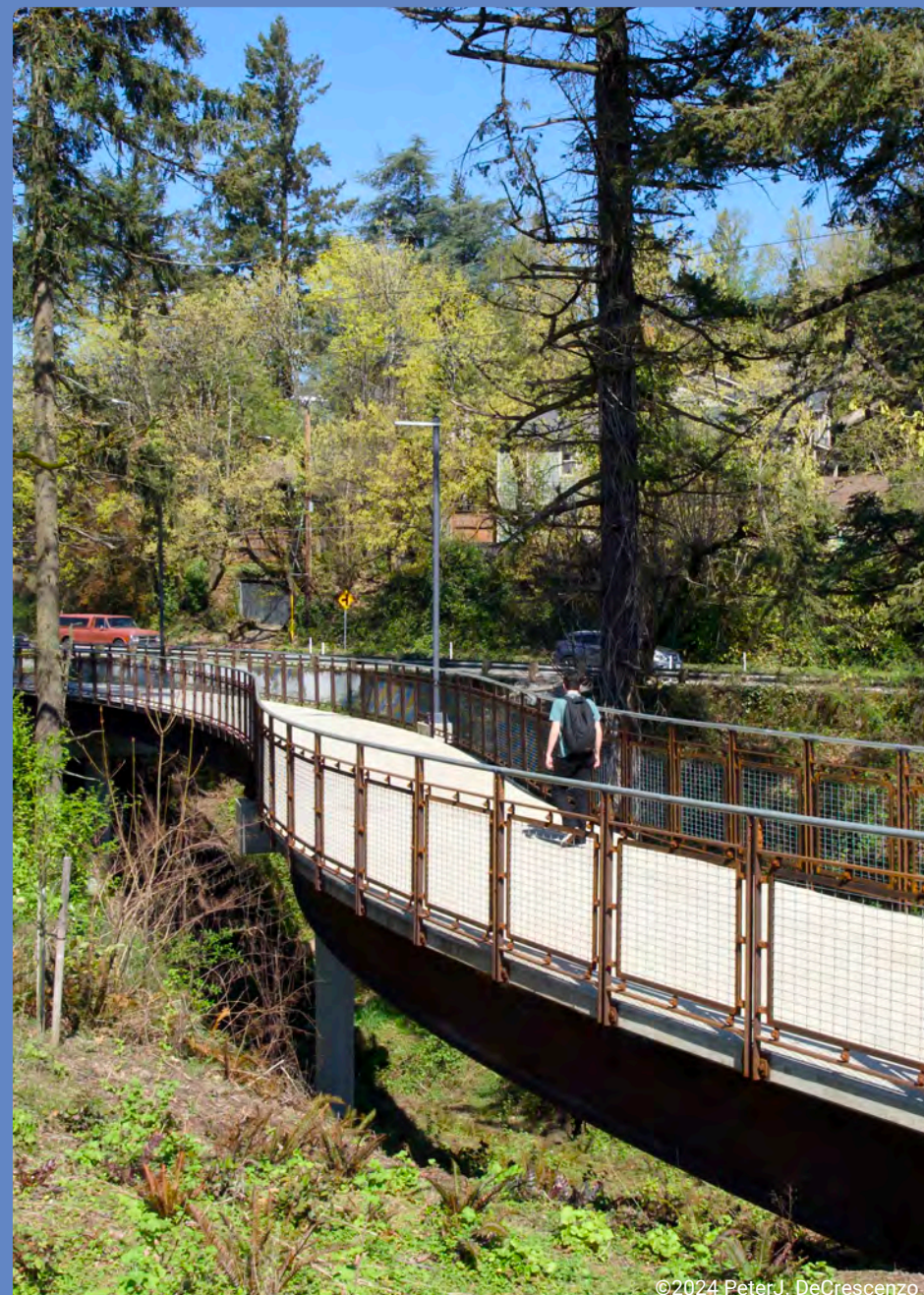
Red Electric bridge
