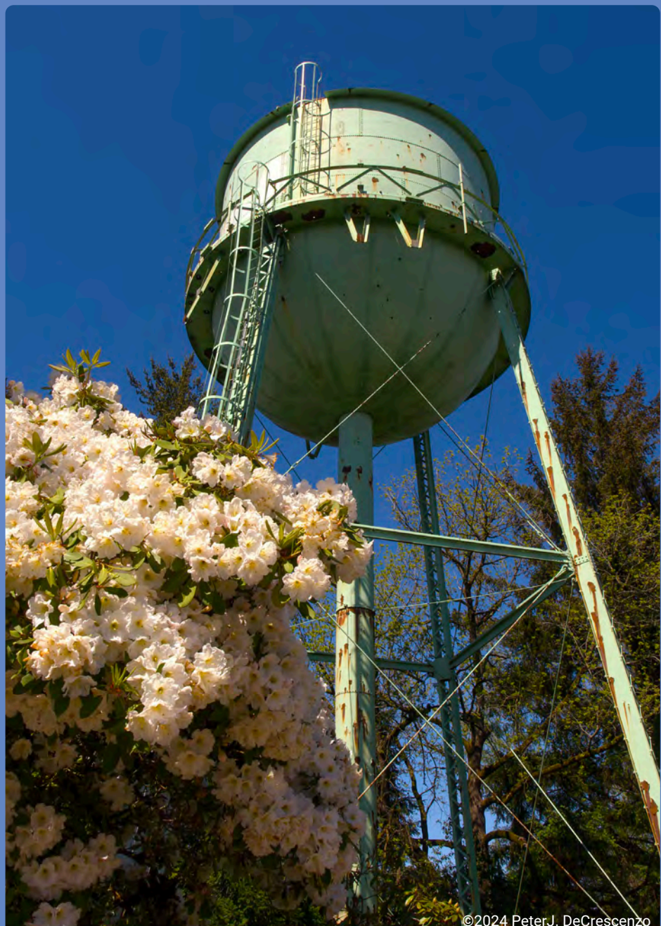
Canby water tower
