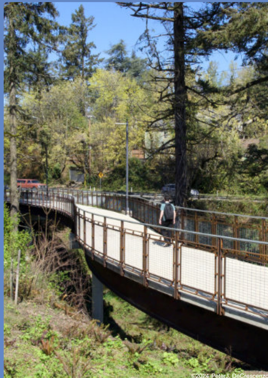
Red Electric bridge
