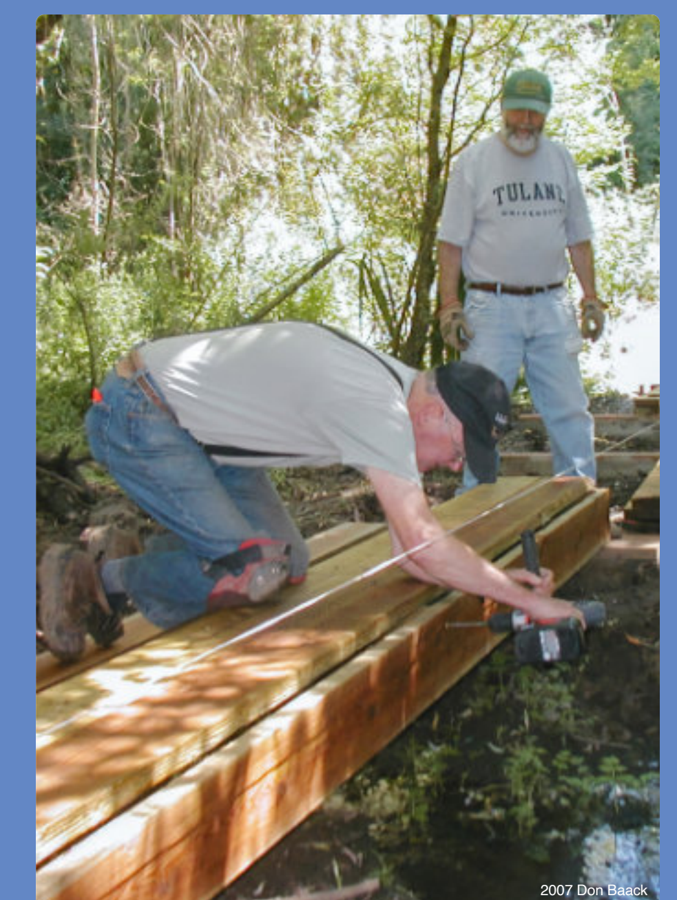
Building the bridge
