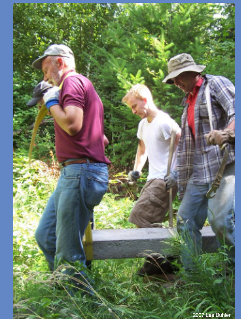
Hoisting a bridge footing
